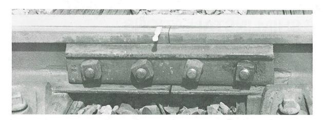
Loosen joint — inspect for cracks — and fit appropriate size of shim to both sides of the joint.
