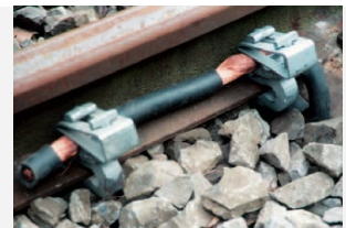
Electrical rail contacts with vibration-resistant cable fixing. Typical arrangement with two clamps and 240mm 2 cable. Ideal for networks with heavy return currents.
