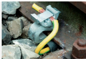
Electrical rail contact with vibration-resistant cable fixing for return current grounding, signal circuits etc.
