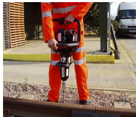
Drilling timber, fixing lag screws/screw spikes between trains
